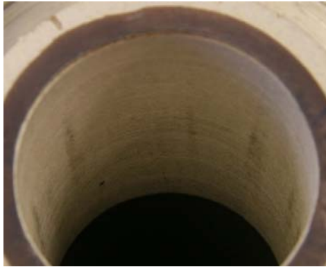
Fig. 17: AvA-Z-ISC material in the oxidation critical zone close to the injector, showing tracks of hot gas attacks.
