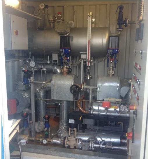
Fig. 2.5 Components of the BoP for pressurised water: expansion tank (top).
