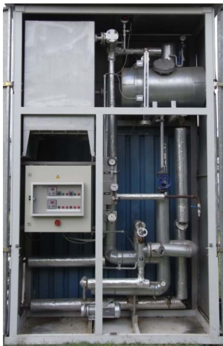
Fig. 2.4 Components of the BoP for DSG: condensing ventilator (top left); steam drum (top right); recirculation pump (bottom centre)
