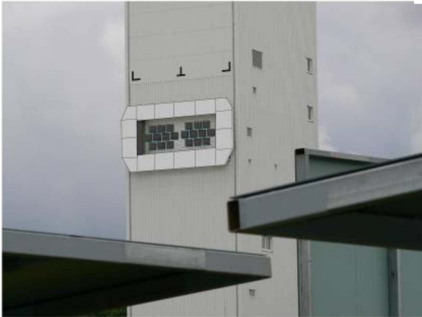
Installation on DLR's Solar Tower Jülich (Artistic View)
