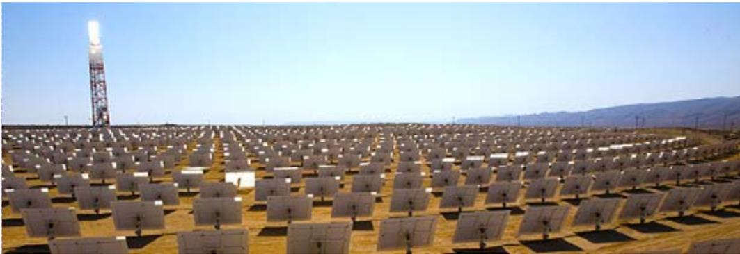
**Figure 1: Solar tower plant (BSE, 2011)**
