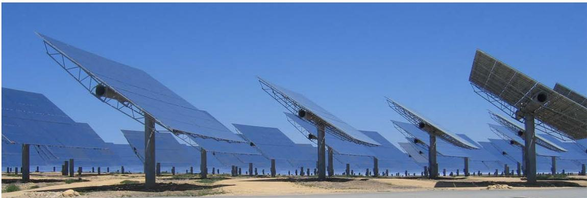
**Figure 3: Heliostats with mirror planes of 120m<sup>2</sup>**
