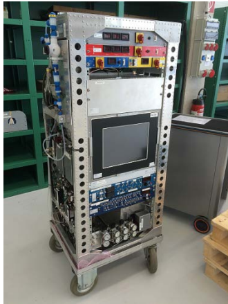
19" cabin racks with instruments
