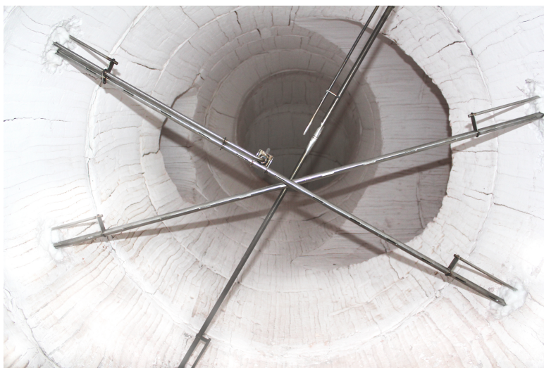
Figure 3.11: Photo of the of the measuring point directly behind the receiver. The photo was taken from the inside of the piping at the STJ. The direction of air flow follows the line of sight. In the background the splitting towards emergency vent, storage and steam boiler (left to right) can be seen.
