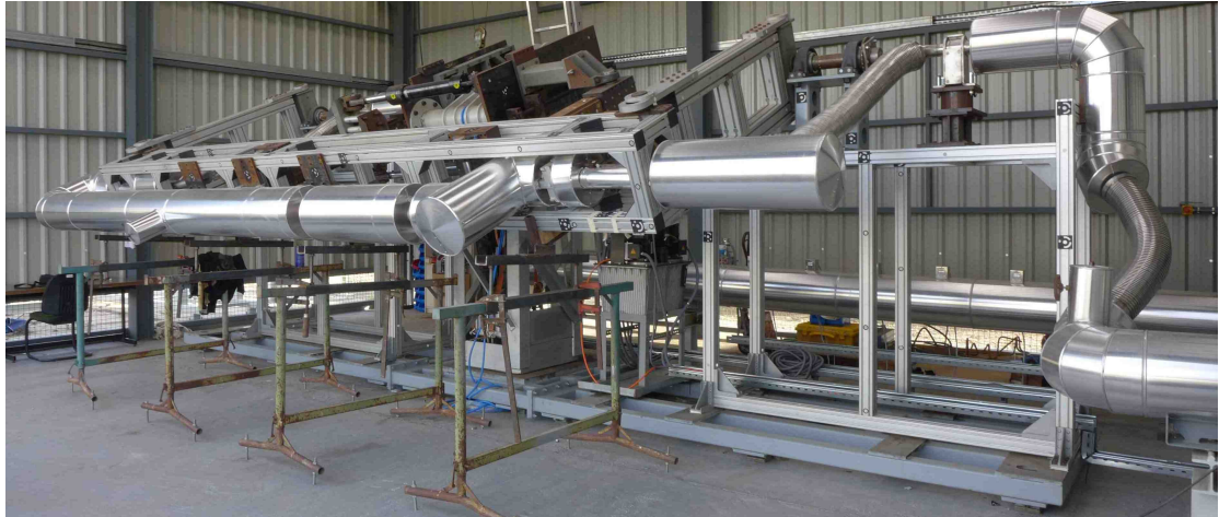
Figure 2.2: The main assembly as built including insulation and REPAs with the traverse still resting on additional supports at stow position.
