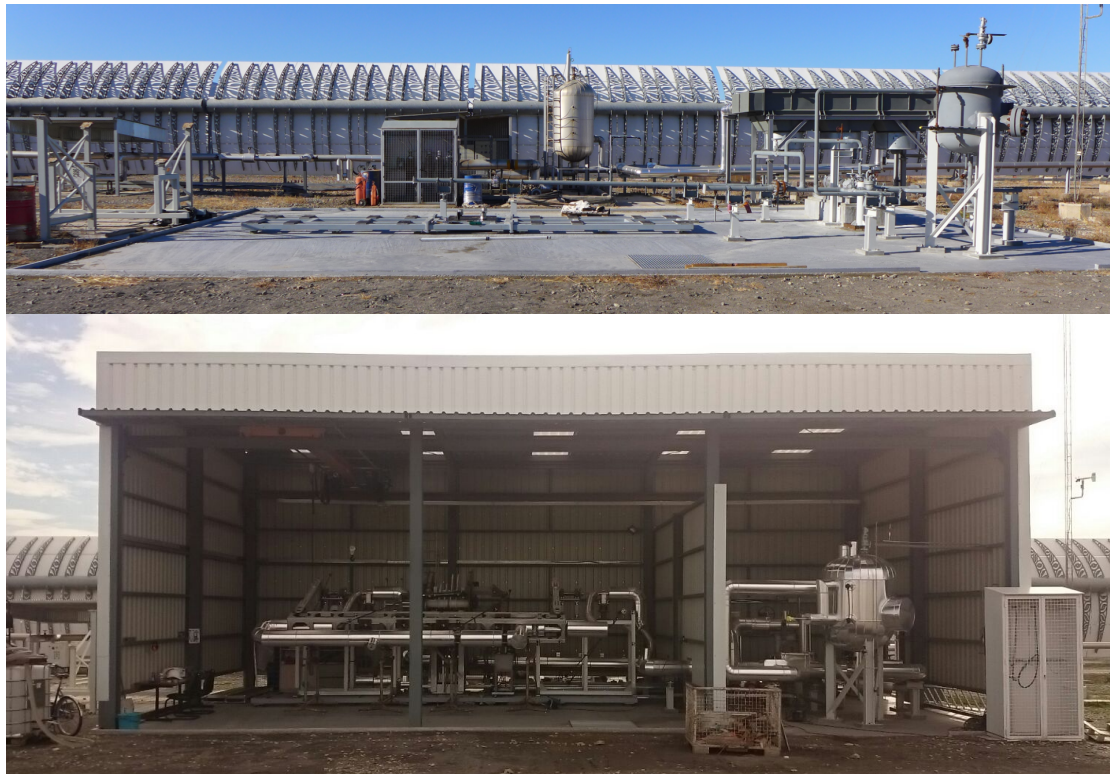
Figure 7.1: Top: REPA test-rig in June 2016, bottom: January 2017
